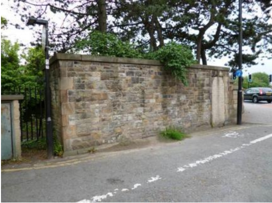
Stone-built former public lavatory attached to Penny Street Bridge
