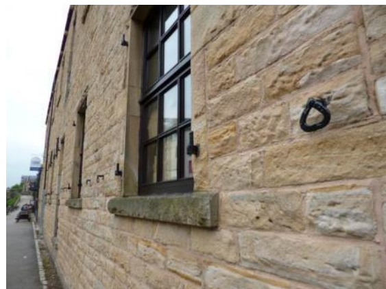
19 th century iron features on canal-side warehouses
