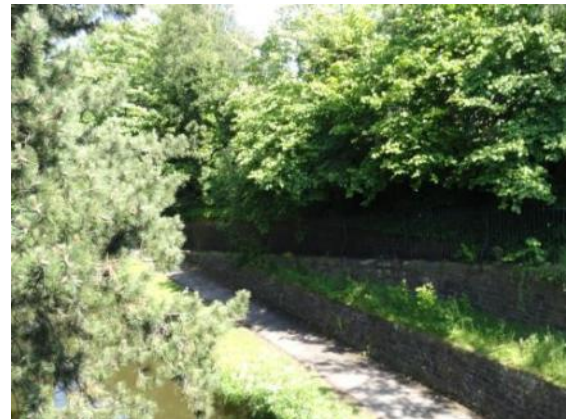
Heavy vegetation in the canal corridor
