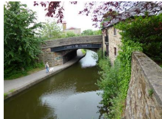
The Nelson Street canal bridge, built 1876 by Joseph Clayton
