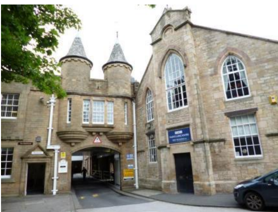
The 1899 entrance block and former Baptist chapel, 1872
