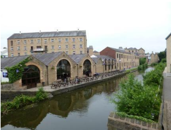
White Cross Mills from the George Street canal bridge
