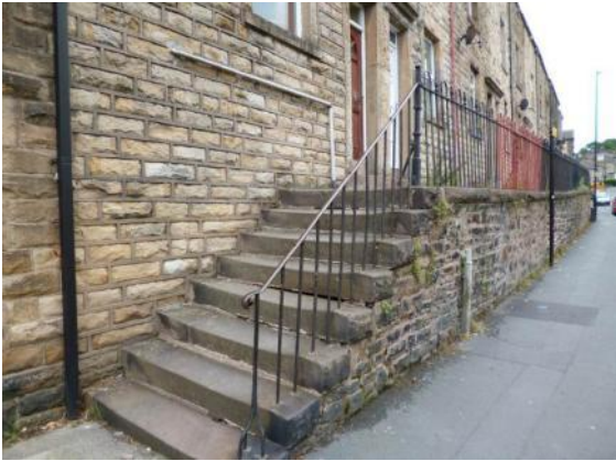
Steps with 19 th century iron railings, Moorgate.
