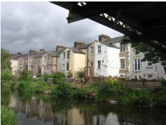
Gabled outriggers face the canal, west side of Wolseley Street
