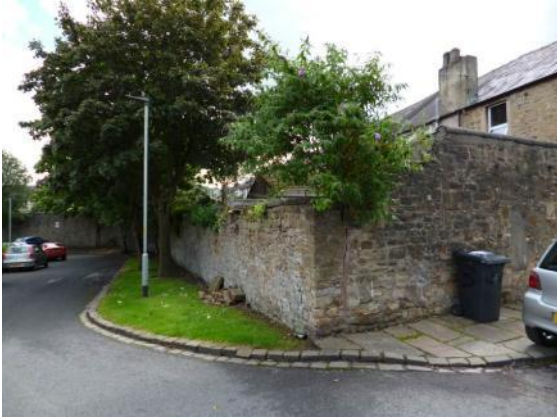
Rear stone walls to yards west of Nuns Street
