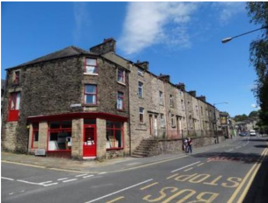
Frontage on Moorgate (showing steps and raised pavement to front doors)
