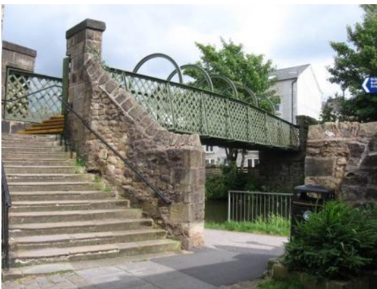
1882 canal footbridge, Shaw Street
