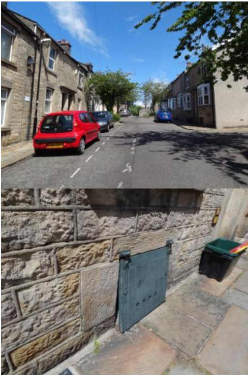
Trees on De Vitre Street; Stone flags and a retained coal hatch to a property
