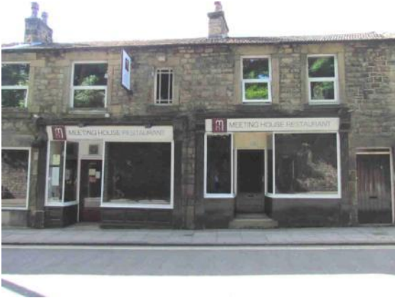
Late 18 th Century buildings on Meeting House Lane with inserted shop-fronts and altered windows
