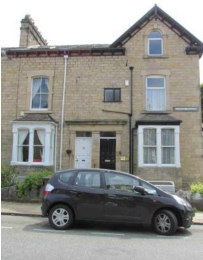
Square bays and gables
