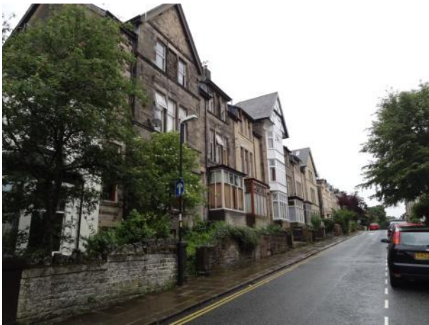
Dramatic change in level within the terrace. (Regent Street)
