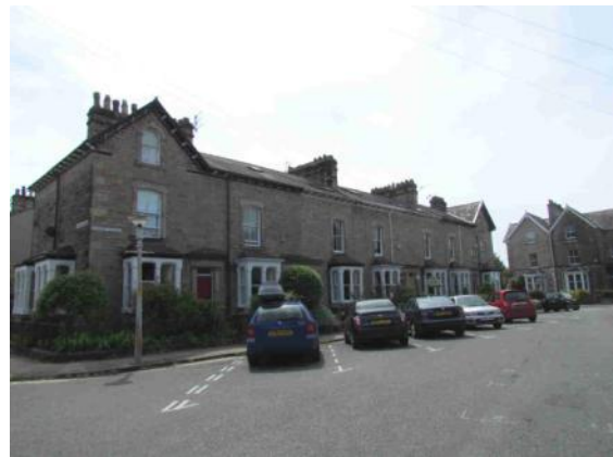
Gabled terrace houses on Lindow Square, 1870s
