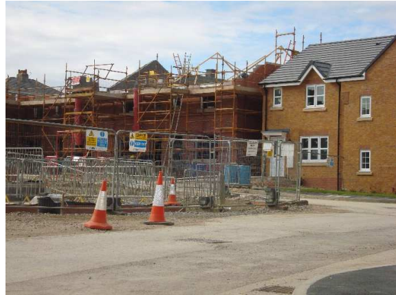
Figure 8 – New housing development within the District
