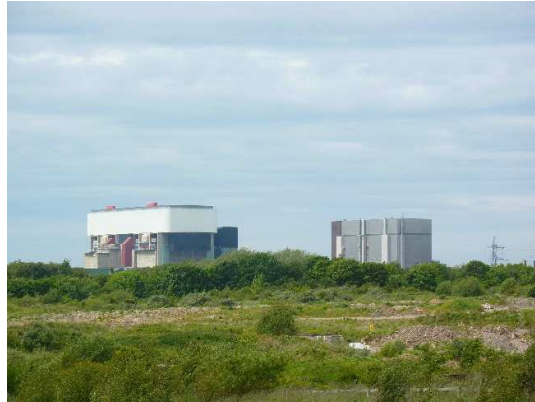
Figure 5 – Heysham Nuclear Power Station
