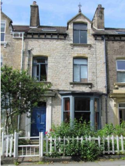
Replacement upper floor windows
