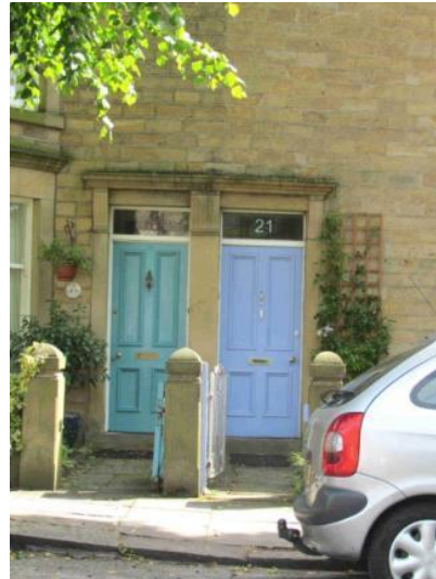
Paired doors with panelled doors
