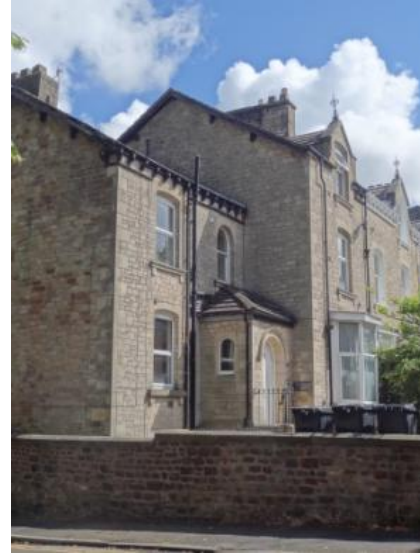
Terraced houses on Westbourne Road
