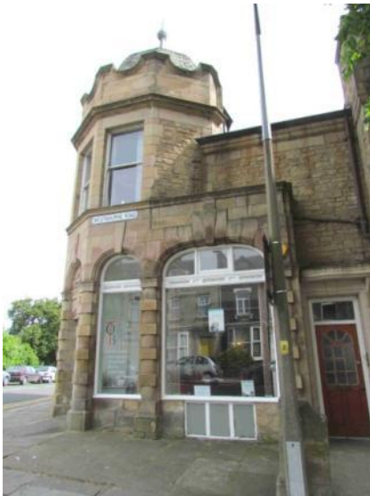
Converted Edwardian Co-operative Shop at 1 Westbourne Road, by Paley & Austin
