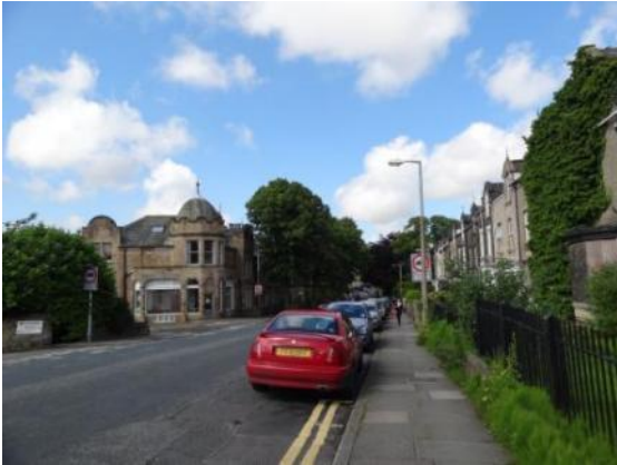
The former Co-op building helps to define the gateway to the area from the east.
