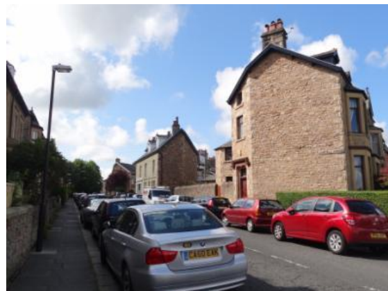
Irregular house type on corner plot on Ashfield Avenue
