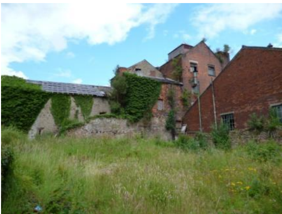
Former brewery buildings awaiting repair and a new future
