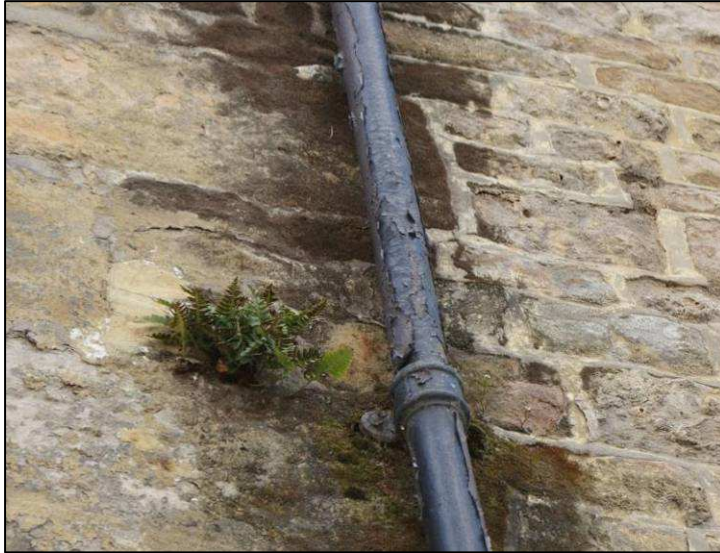
Staining, algal and vegetation growth caused by leaking and unmaintained rainwater goods
