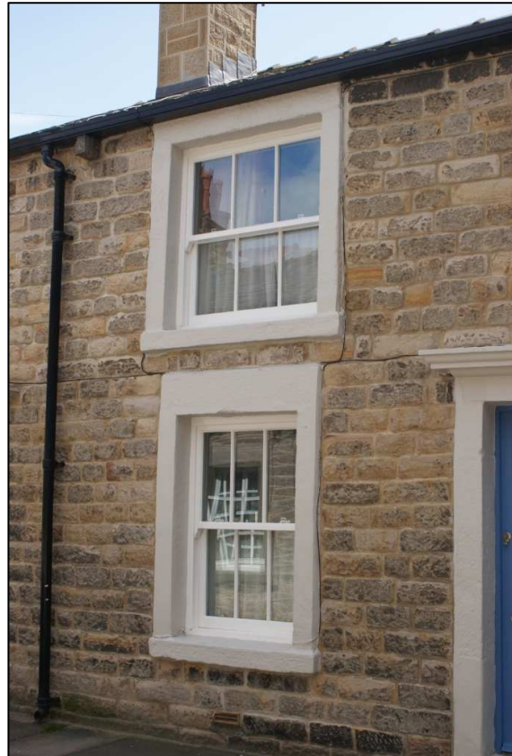
Replacement sash windows
