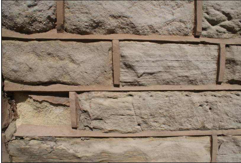
An example of the physical and visual damage caused by inappropriate mortar and pointing
