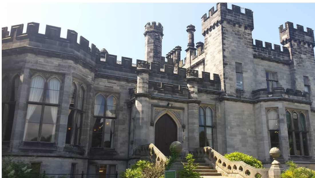
The battlement tower at Ashton Hall (grade I) can be seen to the right in the above photograph
