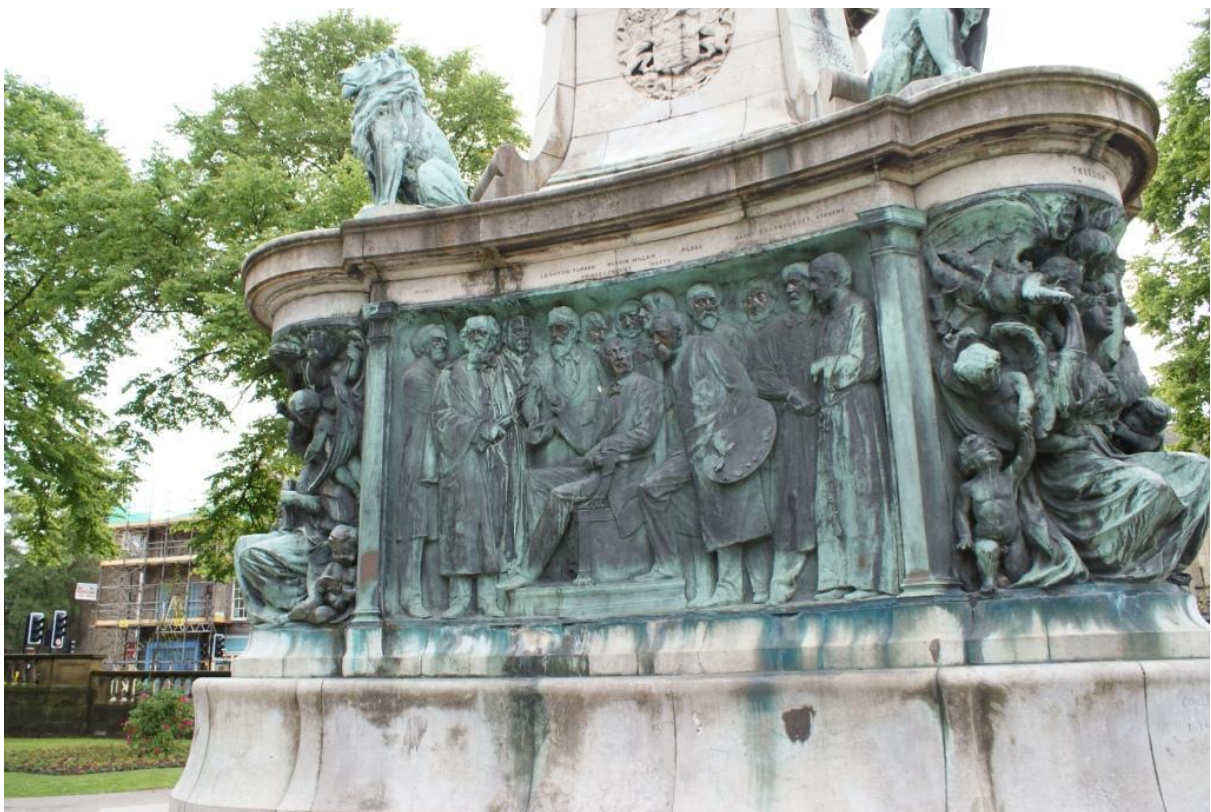
Staining of ashlar
