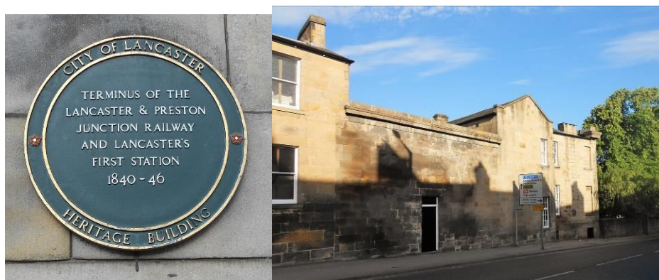
Plaque, above left, found on A6 elevation, above right, of original railway station
