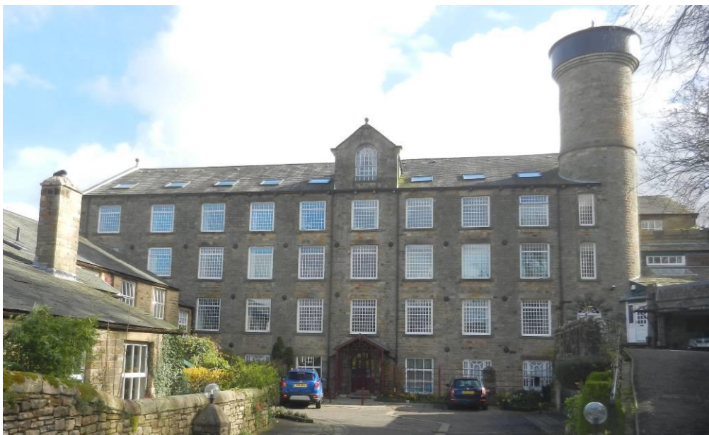
Low Mill, Caton (grade II)
