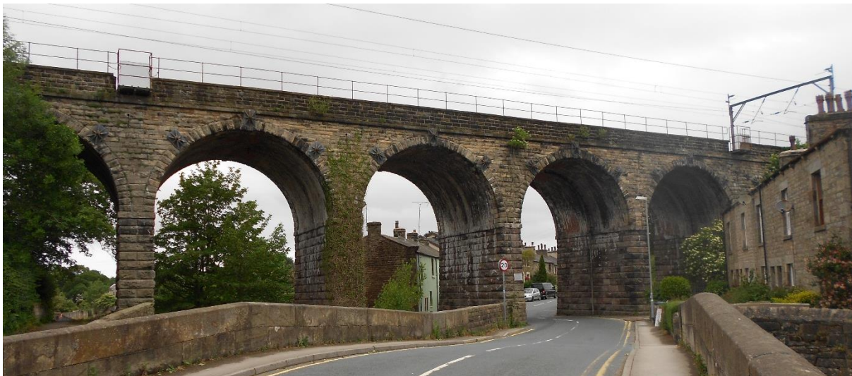
Galgate Viaduct (NDHA)
