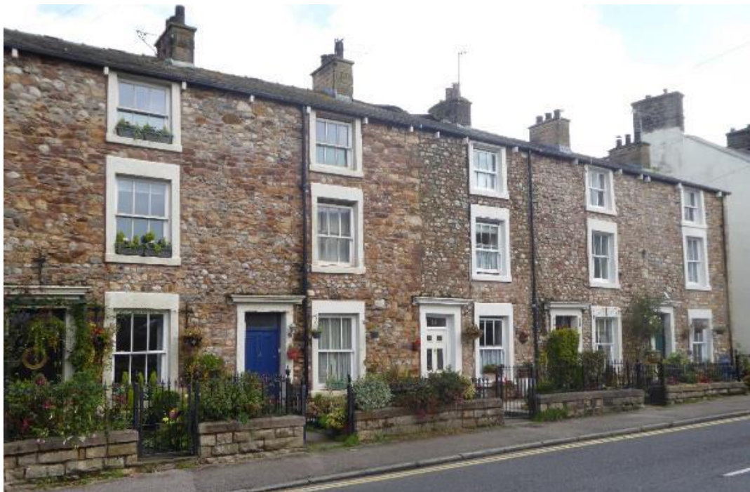
Lord Street Cottages, Morecambe (Article 4 Direction within Morecambe Conservation Area)
