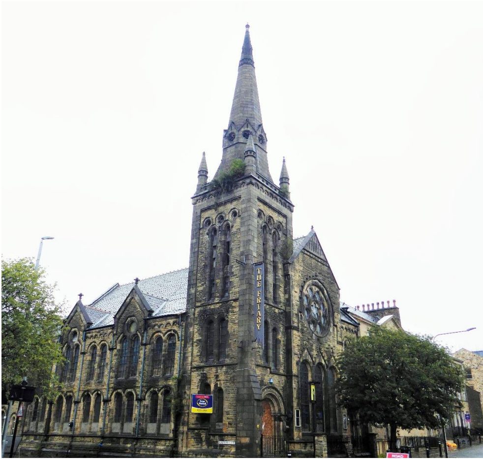
Former Centenary Church, Lancaster (grade II listed)
