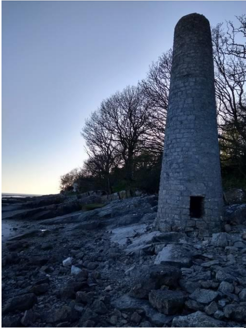
Jenny Brown's Point chimney (grade II)
