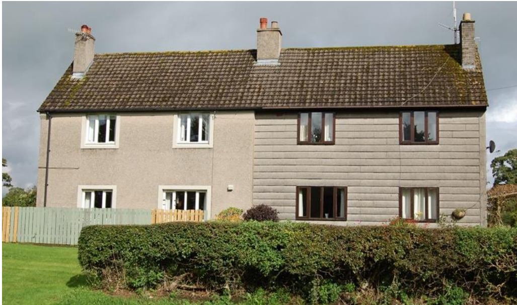
The only original 'Airey' house in Wennington (right). The house next door has clearly since been renovated.
