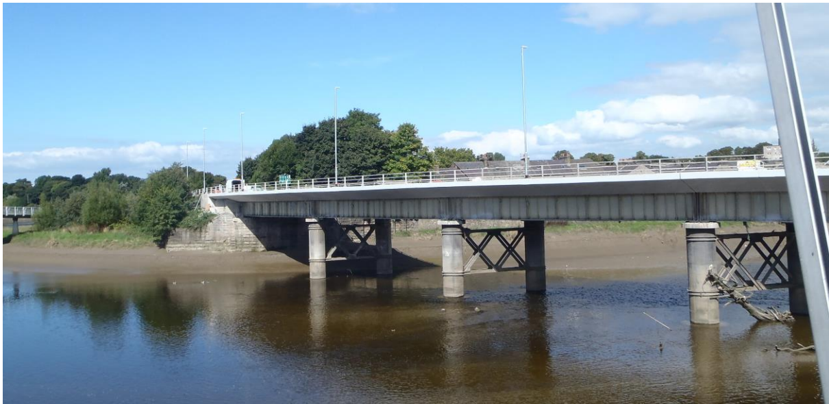
Closed Greyhound Bridge Lancaster
