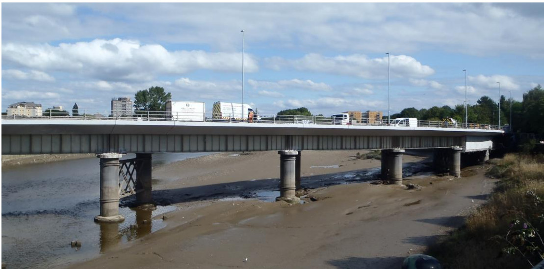
Repair Work to Greyhound Bridge in Lancaster nears an end
