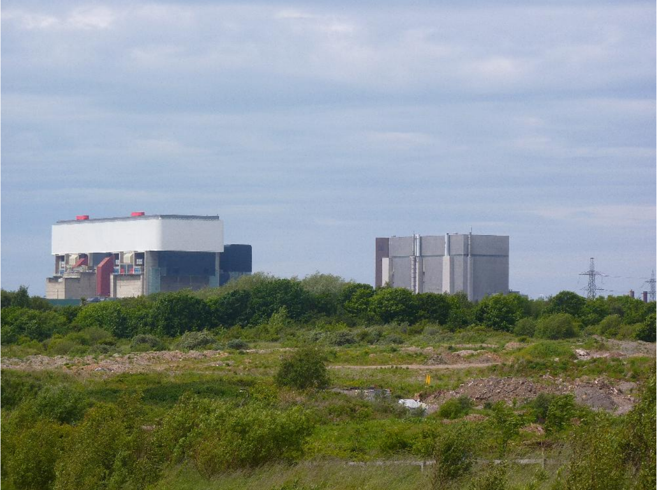
Heysham Power Station
