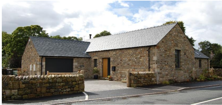
Wenningdale - An example of recent residential development
