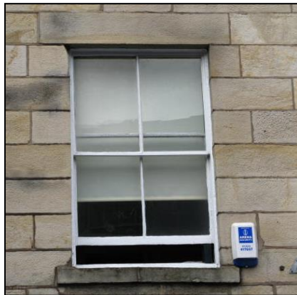
A typical sash window
