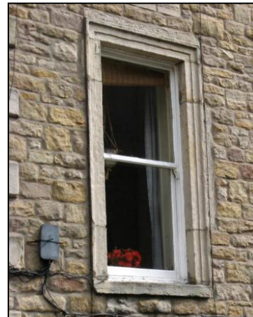
A Victorian sash with sash horns
