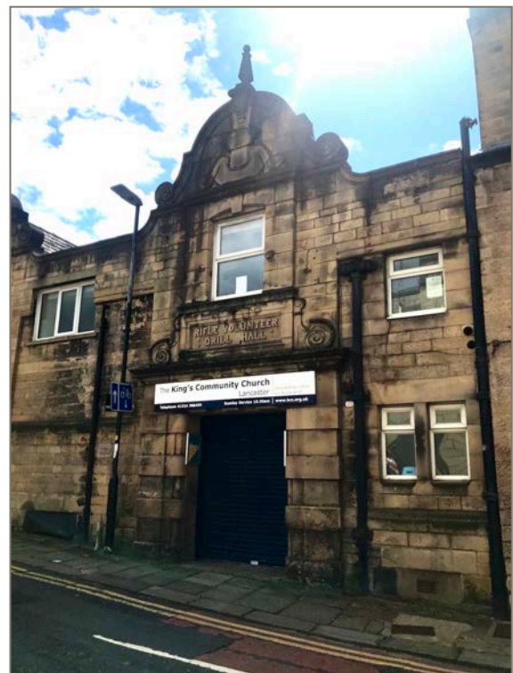
Entrance to the Drill Hall, now the King's Community Church
