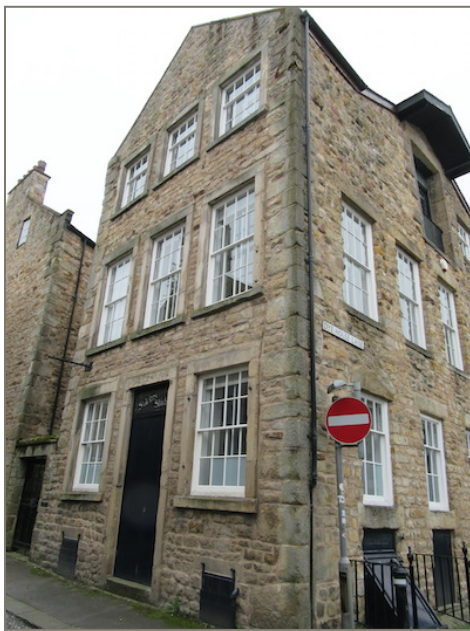
Late C18 warehouse to the rear of 11 Chapel Street.
