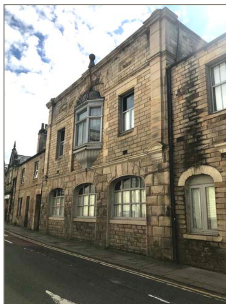
Baroque Revival Phoenix Working Men's Club
