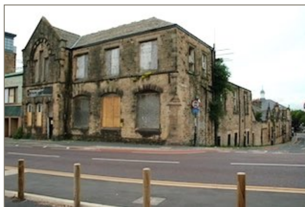
1887 Sunday School Building, St Leonard's Gate, with Phoenix Street beyond
