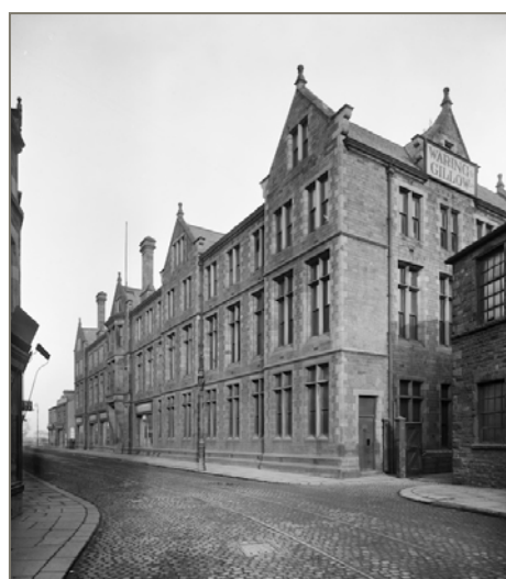
Gillows showrooms, North Road, in 1917 (Historic England ref. BL23741/001)
