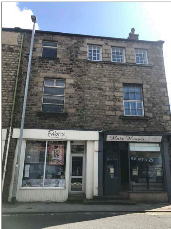
No.s 37 and 39 North Road, originally one house
