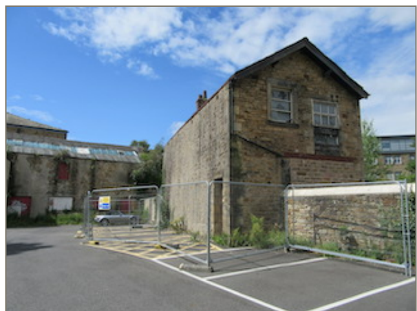
C19 former workshop building, St Leonard's Place
