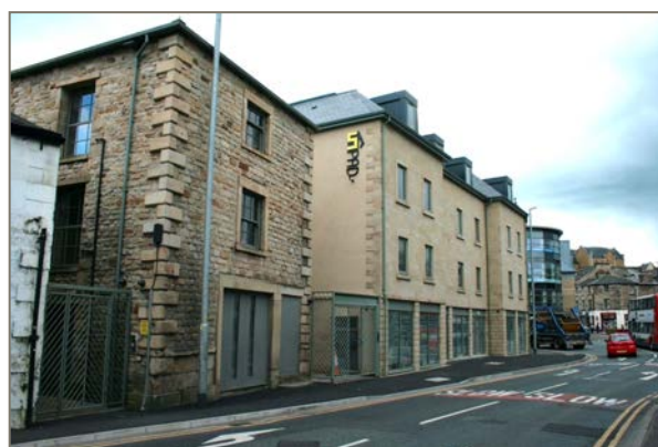
47 North Road in the foreground, with new infill student accommodation beyond
