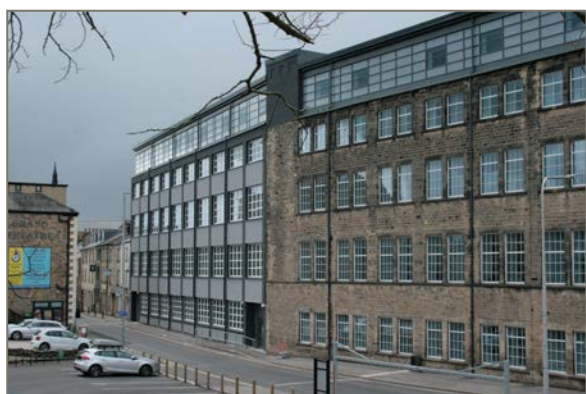
Former Gillows factory, St Leonard's Gate. 1881/2 building with 1920s extension, and recent attic addition.
