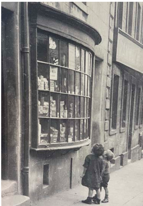
A shop in a former house on St Leonard's Gate, no. 125, next to the Tramway hotel. Taken in 1927, since demolished. Lancashire County Council Red Rose Collection
